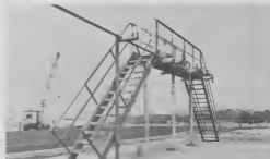
One of the new structures: a loading rack. Uno di e estructuranan nobo: un loading rack.
